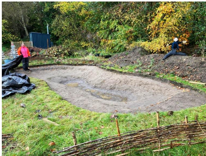
Excavated pond ready for lining
